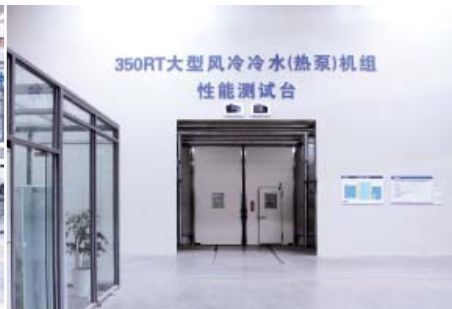
350RT Air-cooled Chiller Test Lab
